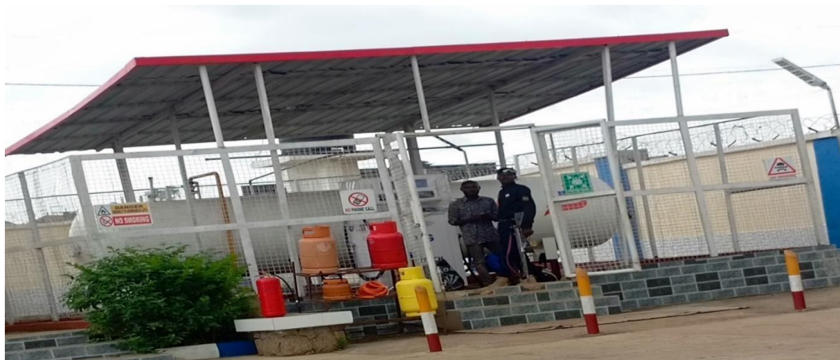
Plate 1: A Protected Retail Point of LPG with Signage Describing Intrinsic Hazard.
