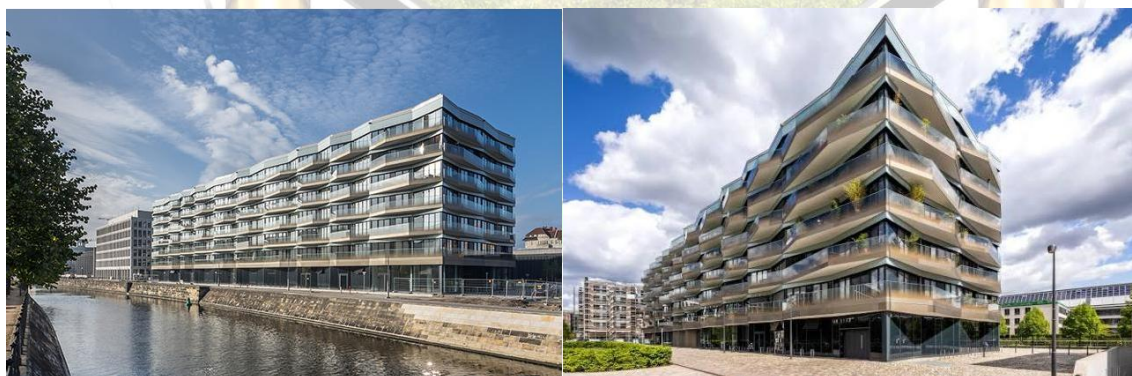
Plates 7–8: The Hamburger Strasse Development, Berlin, Germany, addressing the urban heat island effect and flash floods Source: Alamy (2019). New construction, modern office building, upscale district, Berlin, Germany.
