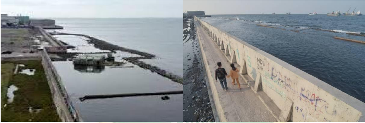
Plates 5–6: The Jakarta Emergency Embankment, Indonesia, addressing land subsidence and tidal flooding Source: Mohd, Z. (2023). Giant wall of sinking city – Jakarta.
