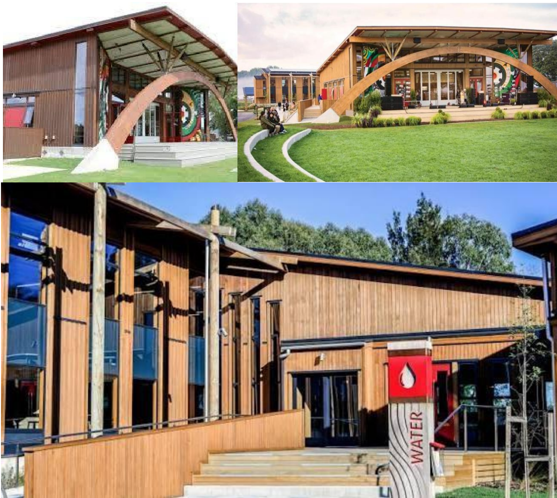
Plates 14–16: Te Kura Whare, Ngāi Tūhoe, New Zealand, designed to address severe storms and power outages Source: Radio New Zealand (2018). A people build a house and a house builds a people.
