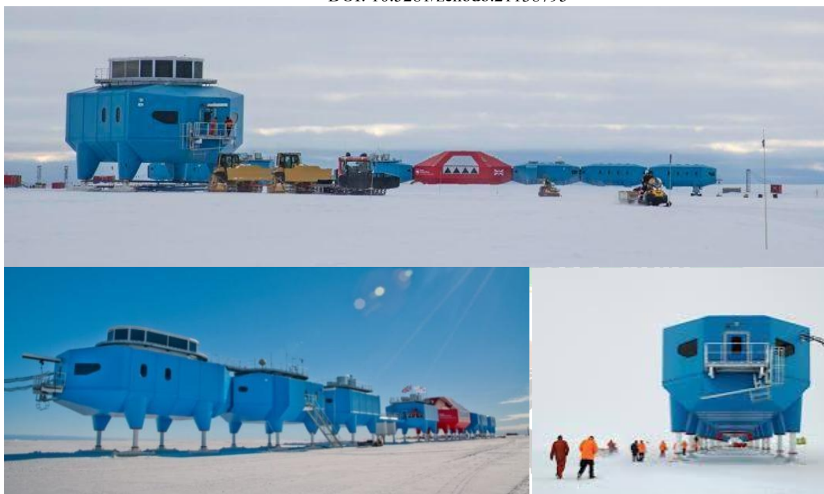
Plates 17–19: The Halley VI Research Station, designed and built to address extreme cold, snow accumulation, and shifting ice shelves
